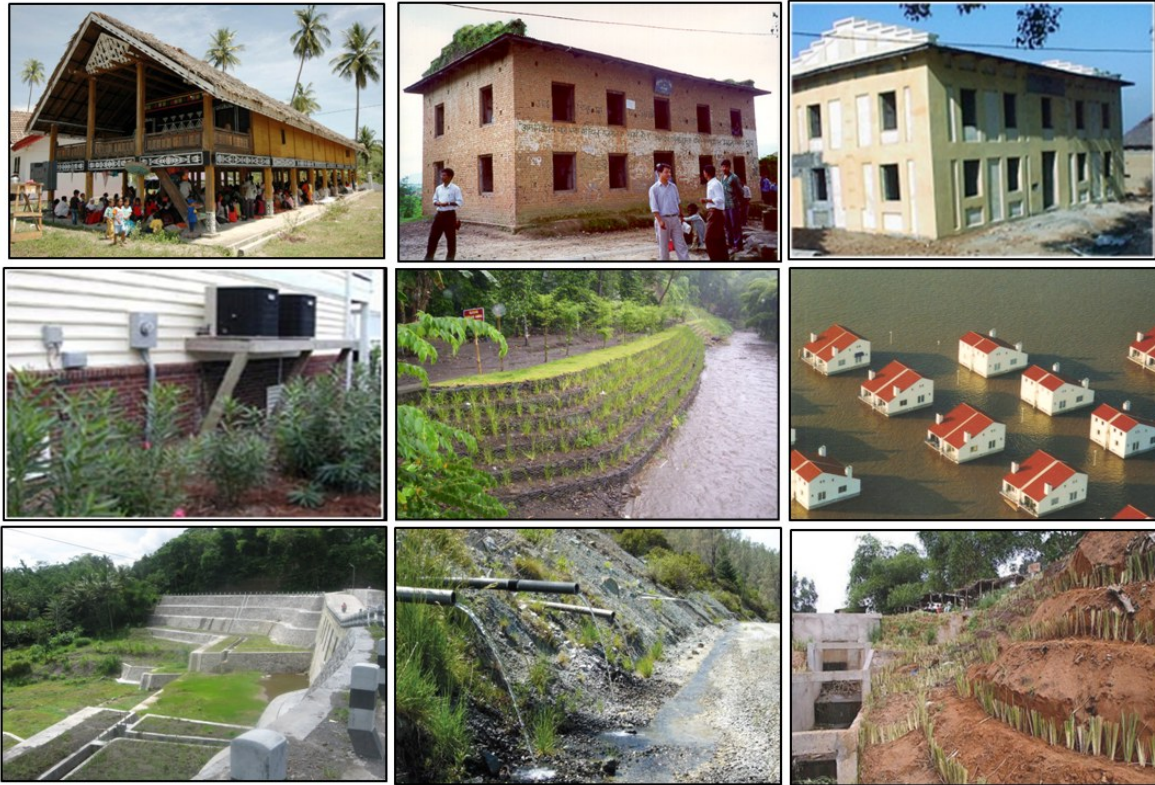
Figure 7.22: Examples of structural mitigation measures. Above: Raised community centre (tsunami hazard), and school retrofitting (earthquake hazard). Middle: raised electrical connection, gabions with vegetation for flood control and floating houses (flood hazard). Below: Retaining walls, slope drainage and biological engineering (landslide hazards)
