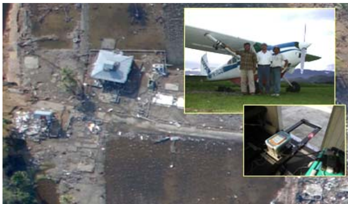
Figure 2.25: Damage mapping using small format aerial photography Aceh tsunami disaster (Photos: B. Widartono, UGM, Indonesia)
