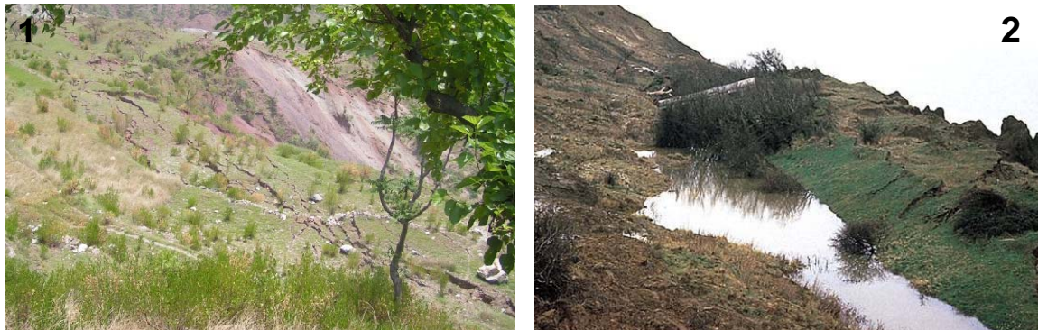
Fig. 3.1.10: precursors of landslides. Image 1: multiple crack array in the area of Upper Killha, Azad Kashmir; failure of these slopes in the forthcoming monsoon looks to be very probable. Image 2: springs on a slope after heavy rainfalls.
