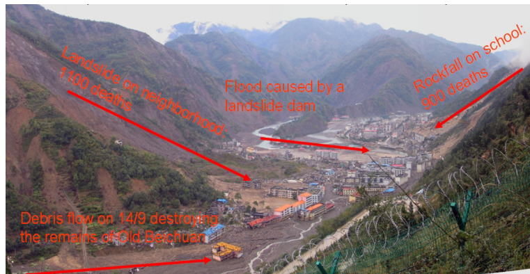
Figure 3.L.1: Illustration of the devastating effects of landslides related to the Wenchuan earthquake in 2008. The city of Beichuan was destroyed by 2 large co-seismic landslides, later on flooded by a landslide dammed lake, and the remains were destroyed later on by debris flows during the first rainy season after the earthquake.
